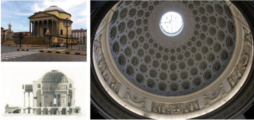
Fig. 9.1 Rosettes under the dome ( Gran Madre di Dio , Turin, Italy). Notes Exterior of Gran Madre di Dio (left top); cross section diagram (left down); dome (right). Sources Tripadvisor (left top); Museo Torino (left down); Vanupied, Photo by Gianni Caeddu (right)
